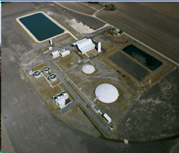
East Williamson County Water System
